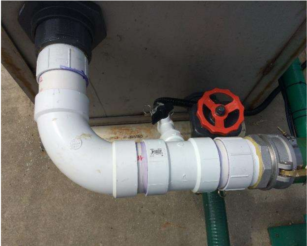
Figure 3.1-3: Scent Line from Collection Tank Gravity Feed to Ramp, 2017
