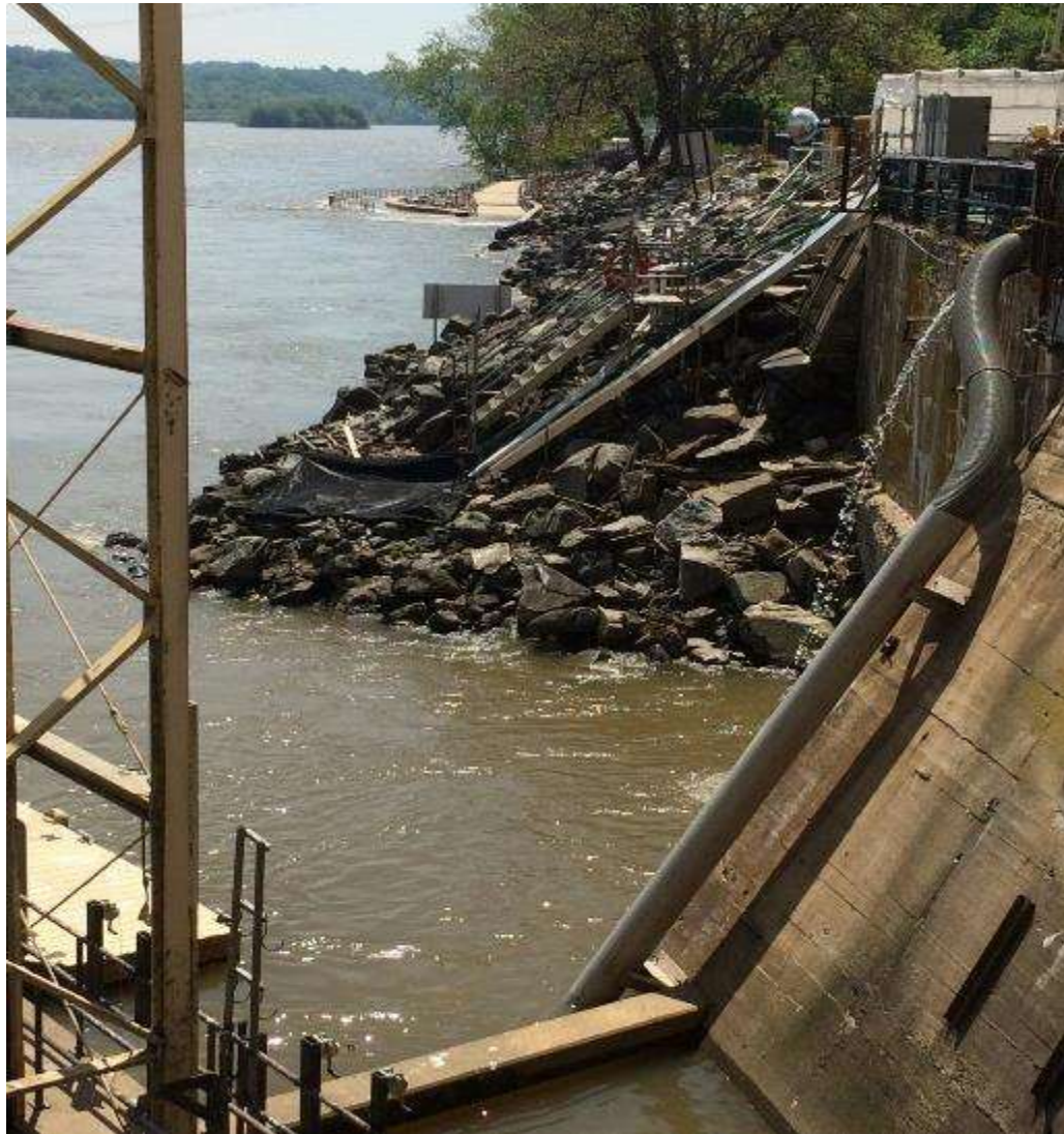
Figure 2.0-2: Location of the Conowingo Eel Collection Facility Just Downstream of the West Fish Lift, Conowingo, MD, 2017
