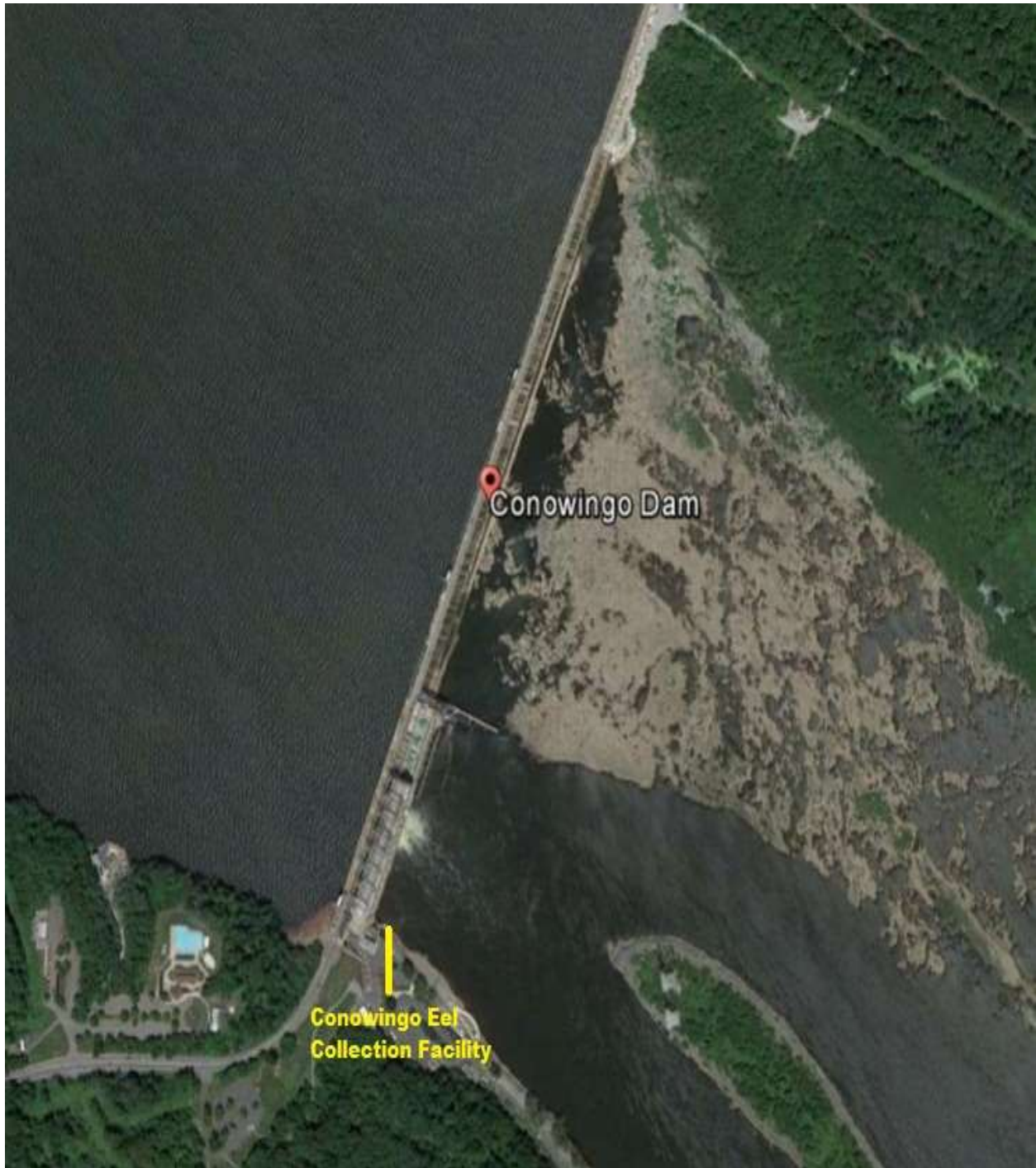
Figure 2.0-1: Location of the Conowingo Eel Collection Facility at Conowingo Dam, 2017
