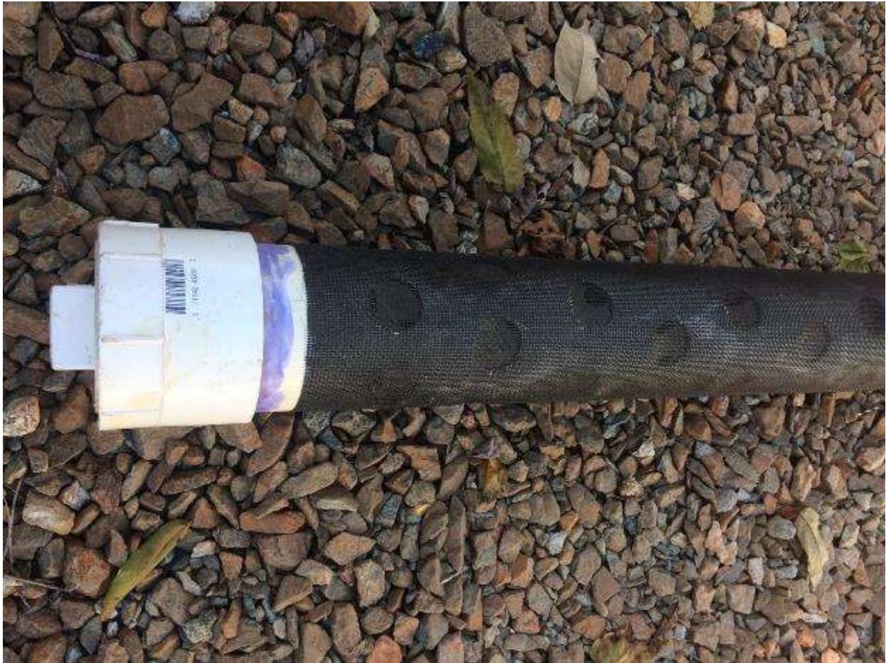
Figure 3.1-10: Screen Drain in Collection Tank, Conowingo Eel Collection Facility, 2017
