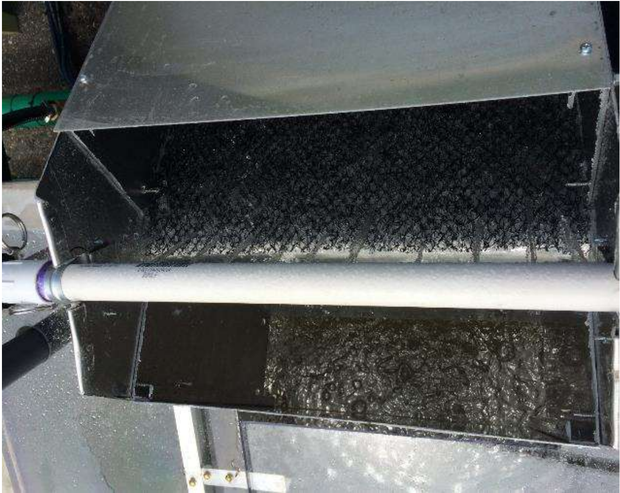
Figure 3.1-2: Attraction flow from Spray Bar, Conowingo Dam, 2017
