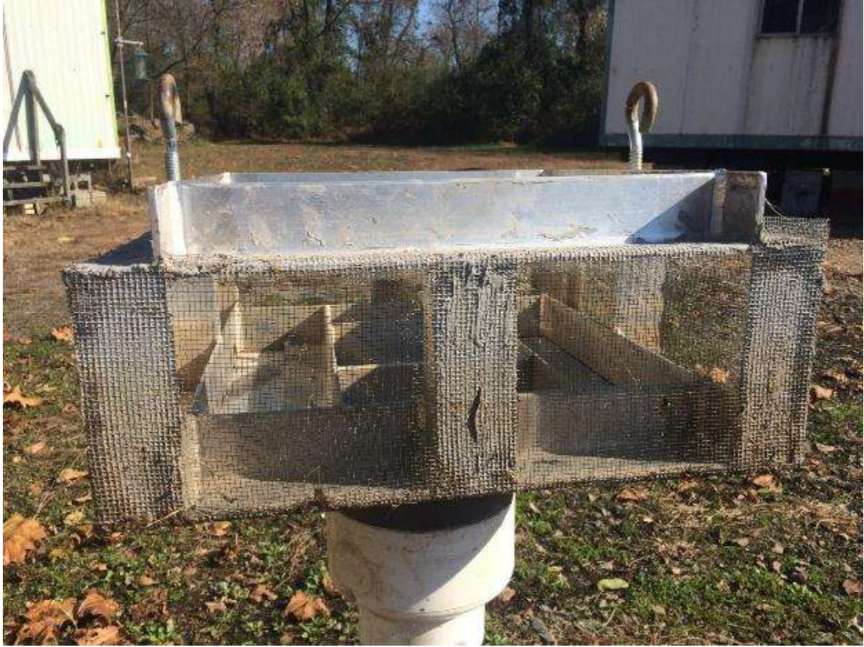
Figure 3.1-12: Screened Drain for Holding Tanks, Conowingo Eel Collection Facility, 2017
