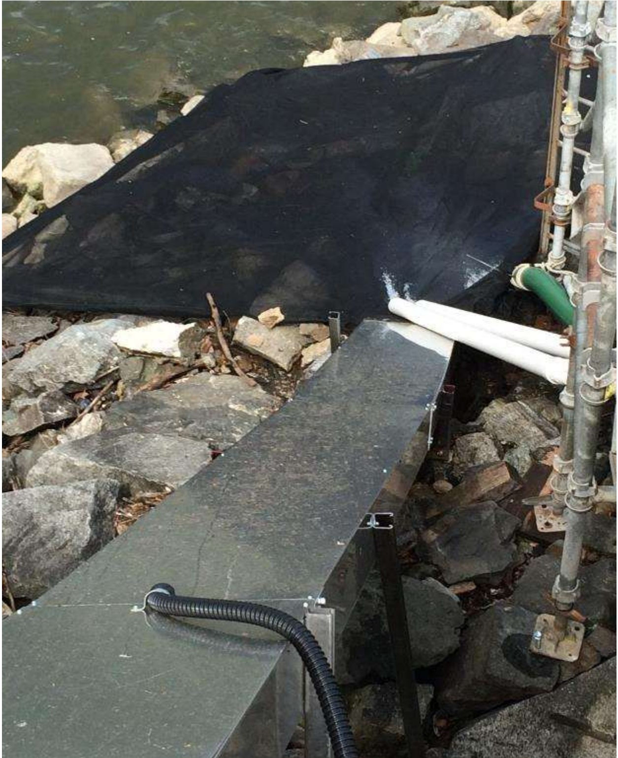
Figure 3.1-8: Cover Over Eel Ramp and Rip-Rap to Protect Eels, Conowingo Eel Collection Facility, 2017
