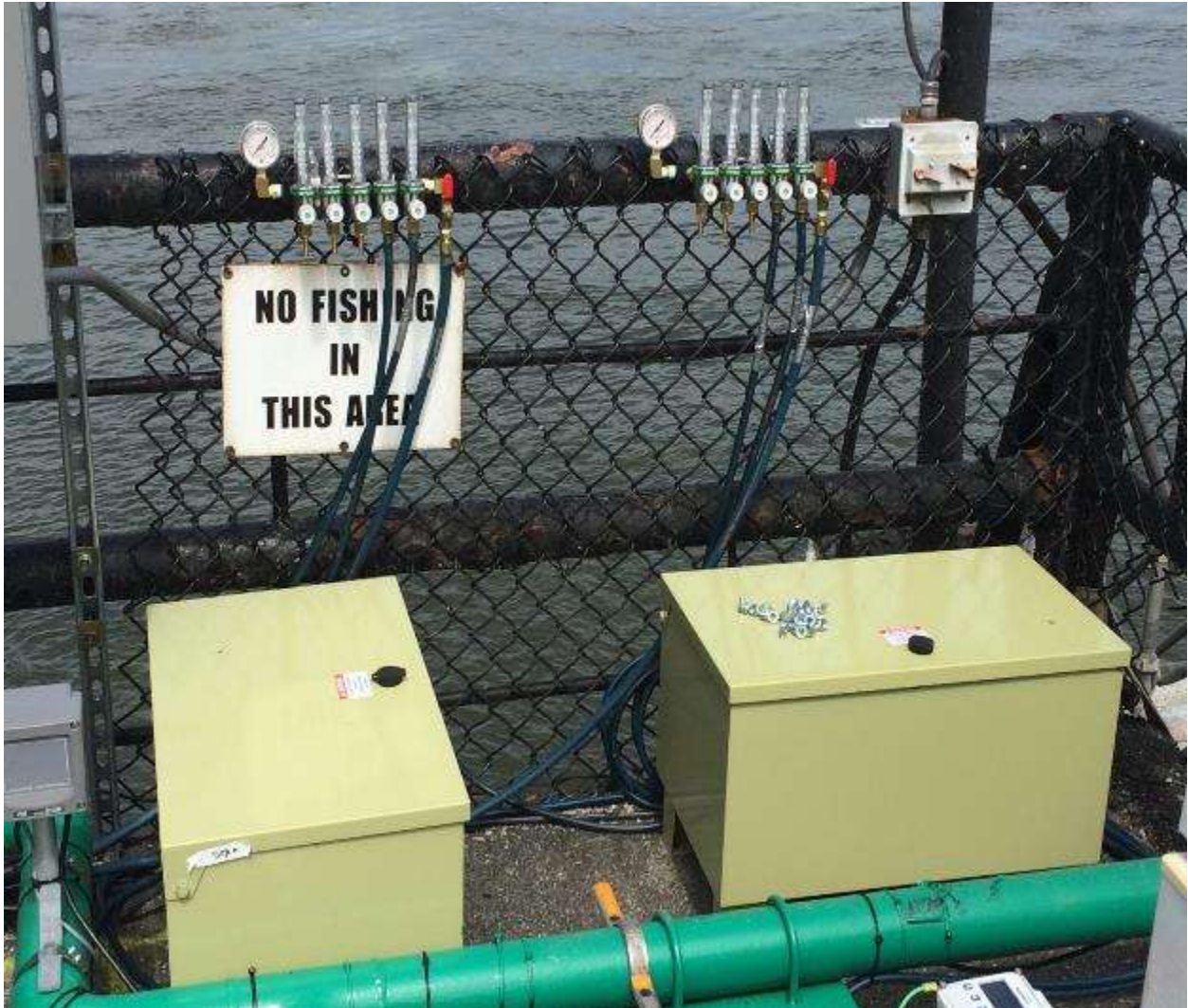
Figure 3.1-5: Air Blower Oxygen Manifold for the Conowingo Eel Collection Facility, 2017
