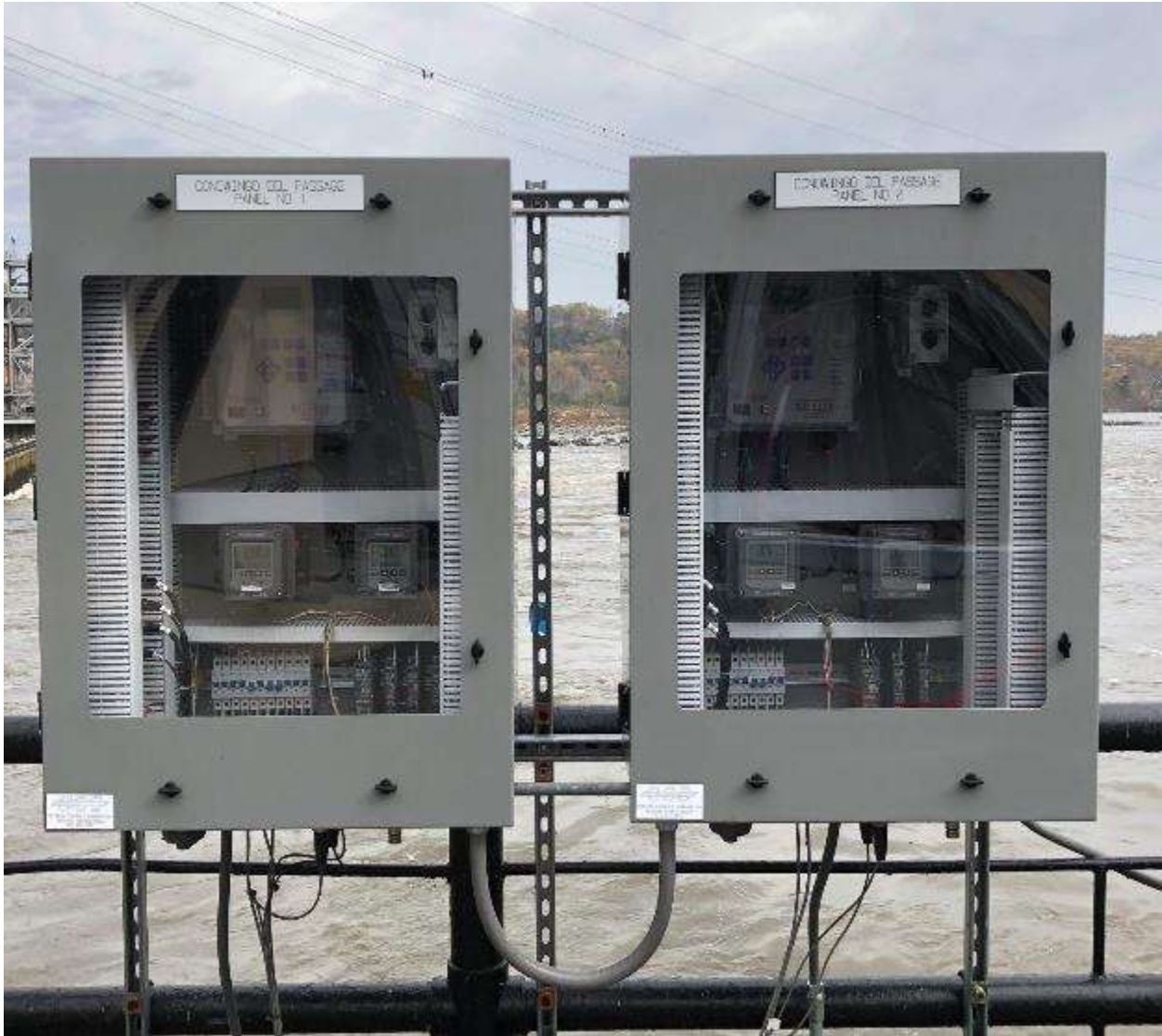
Figure 3.1-4: Control Panel for Read-outs, Conowingo Eel Collection Facility, 2017
