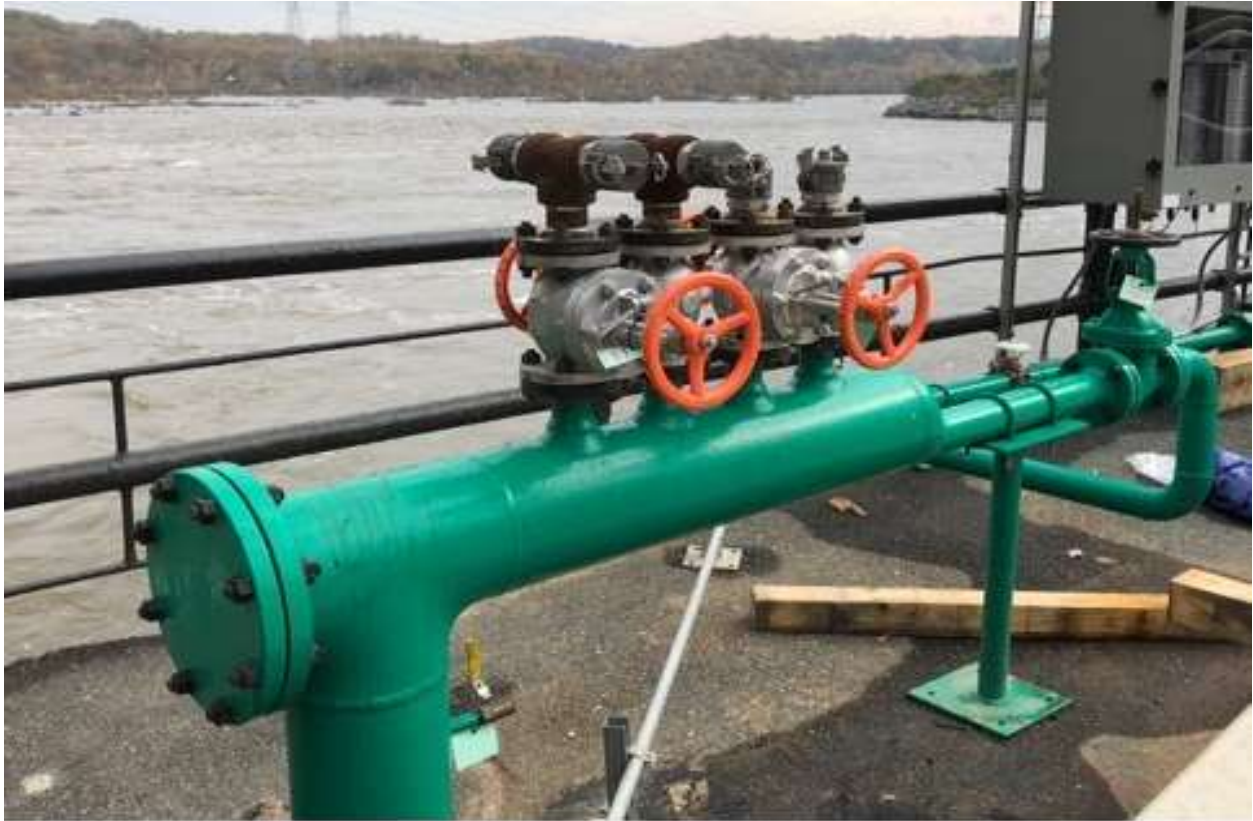
Figure 3.1-1: Gravity Feed Water Line for Conowingo Eel Collection Facility, Conowingo Dam, 2017
