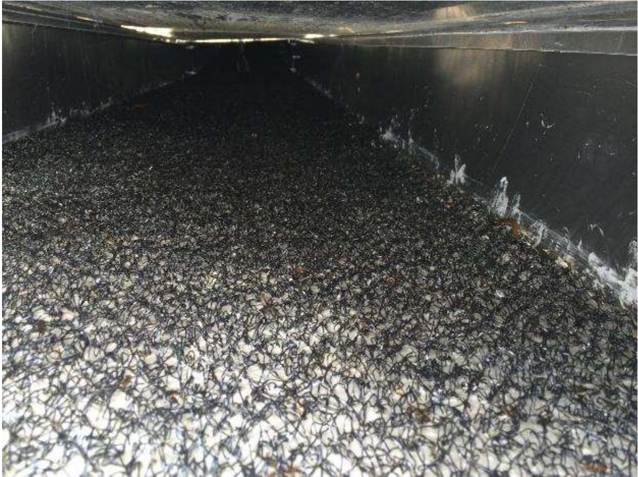
Figure 3.1-7: Juvenile Eel Ramp and Substrate (Enkamat) at the Conowingo Eel Collection Facility, 2017
