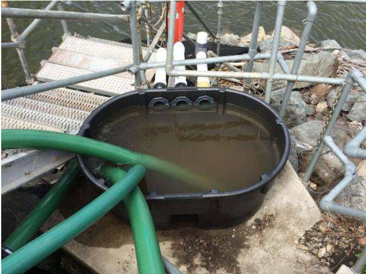
Figure 3.1-13: Over Flow Tank, Conowingo Eel Collection Facility, 2017
